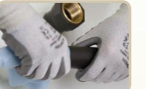
**6** **Clean the parts to be welded**, first female then male, using CLEANER+. Use a clean, lint-free piece of cloth. Leave to dry or wipe dry using a soft, lint-free piece of cloth.
